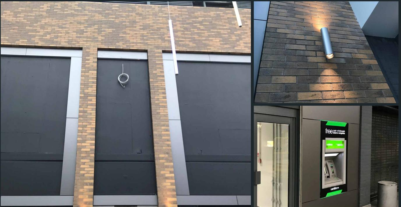
**Trespa cladding is available in a wide range of different finishes and colours which meant that the architect did not have to compromise on the final look. The finish chosen for this project was a plain grey panel, fitted using the BBA certified Nvelope support system, to frame the large advertising screens around the centre.**
