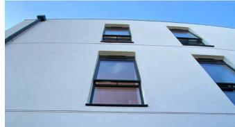
Main Contractor Darwin Group, who we've worked with in the past, engaged us to install the insulated render system and the decorative Rockpanel cladding which had been specified for the coloured areas at the front of the building. Rockpanel is a sustainable cladding option created from volcanic rock and is available in a broad range of colours.
