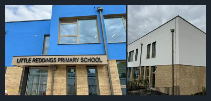
Our scope involved installing the EWI PRO rendering system and Mineral Wool Insulation Slabs. The client specified these insulation slabs for their exceptional acoustic, thermal, and A-rated fire performance.
